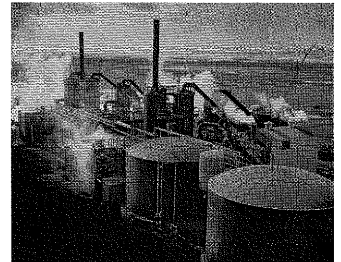
▼ Sulphuric acid production plant, using contact process, furnishes acid for company mill and for other uranium processing mills in the district.
