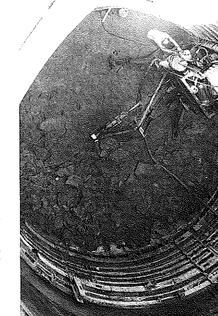
Sand becomes chunks of frozen material under the freezing techniques employed in this shaft.
