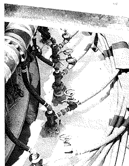
Intricate pipe and valve system surrounding the freeze collar.
