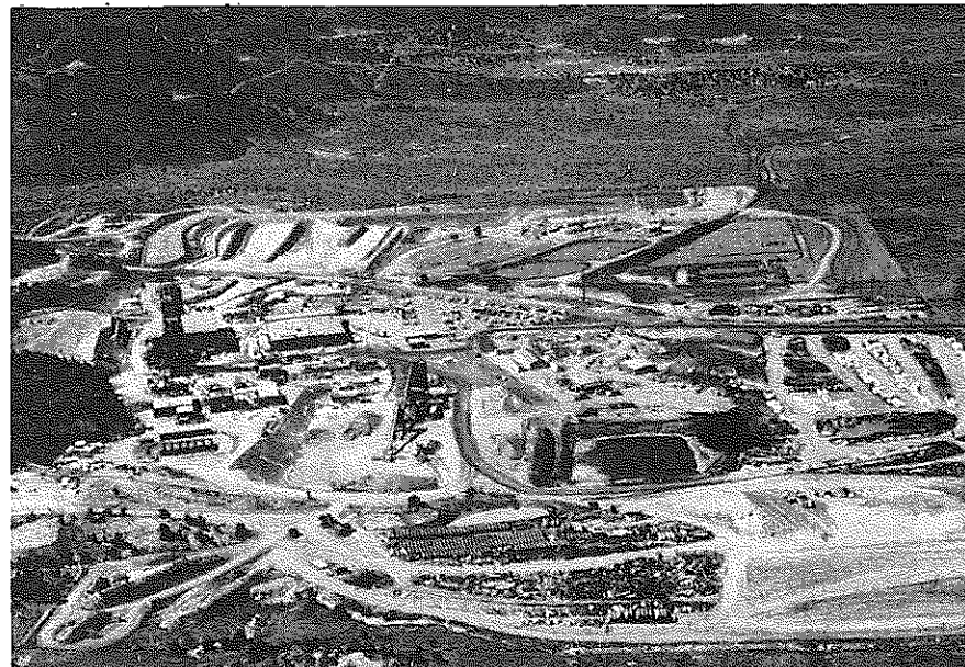
An overview of the Mt. Taylor project, picturing the complexities of the operation and its size.
