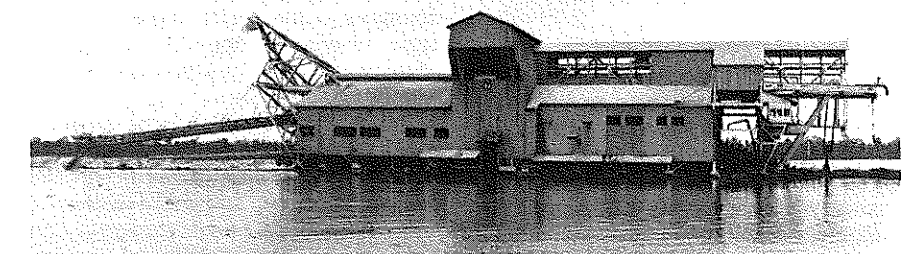
A bucket line dredge mining offshore in Malaysia.
