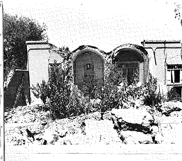
Destroyed home near the Muslim Shrine in Kakh.
