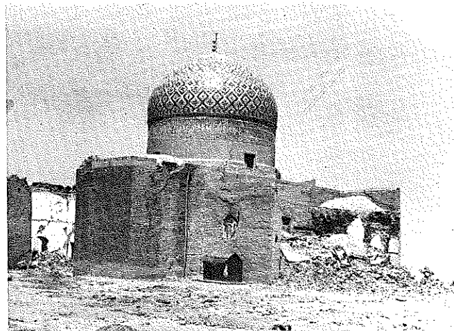
Damage to Muslim Shrine in Kakh.
