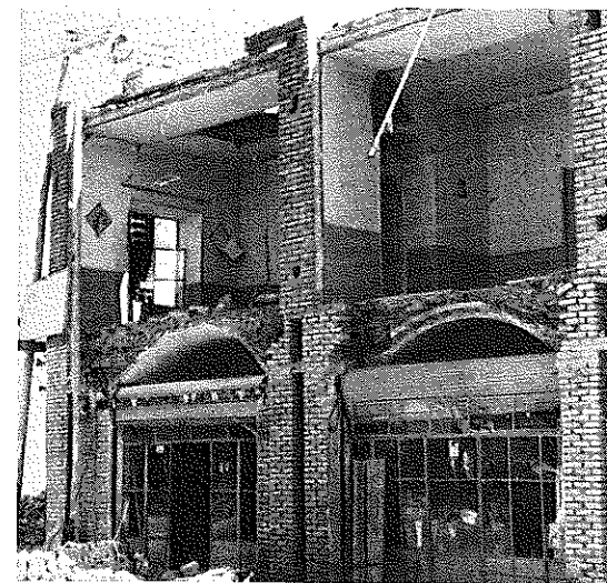
Two-story building damage in Firdous.
