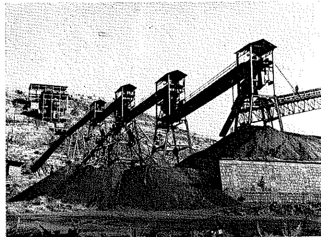
▼ Steel bridge and automatic screen selectors on face of Cerro de Mercado, Durango, Mexico.
