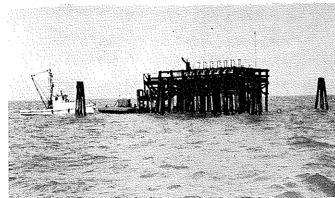
▼ Gas Control and metering platform in Matagorda Bay.
