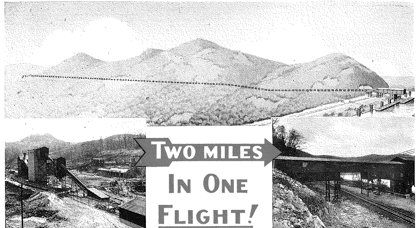
Here coal is prepared in this new blending and washing plant completely designed and built by Link-Belt. From this plant the washed coal is delivered to the tunnel belt conveyor (right side of above photograph) on which it is transported to the river and rail loading station.
