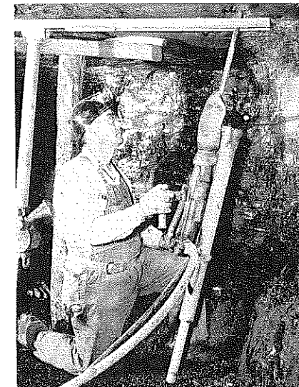
▼ Drilling for placement of C.F. & I. Roof Bolts, Coal Mine, Trinidad, Colorado
