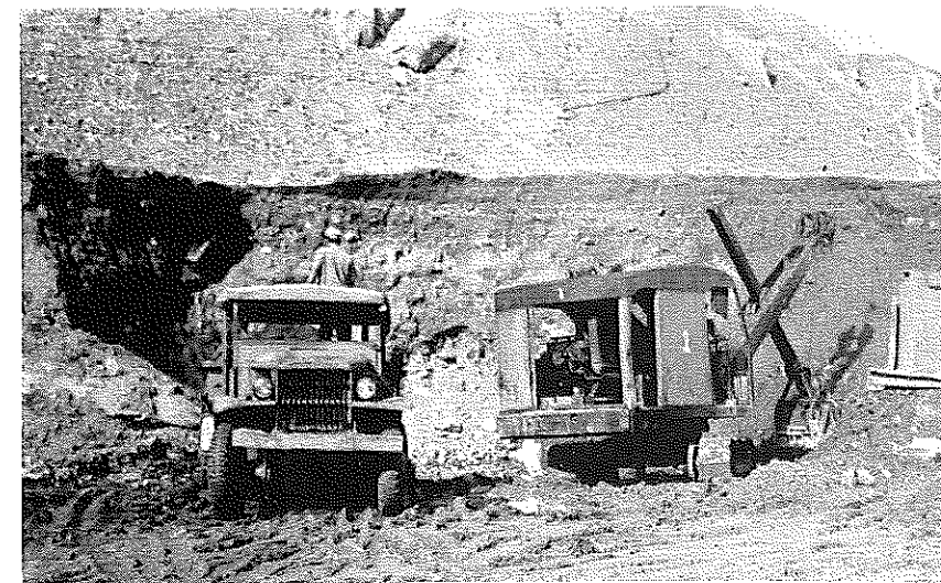
▼ Shovel loading chromite from old dump.
