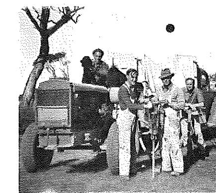
▼ Jackhammer used instead of the intermediate auger where underlying rock is too hard.
