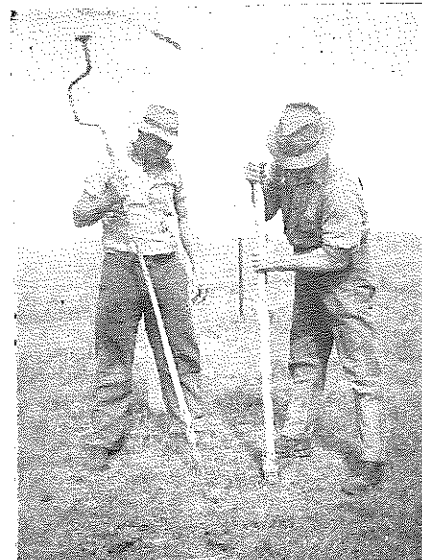
▼ Inserting small casing after using intermediate auger.
