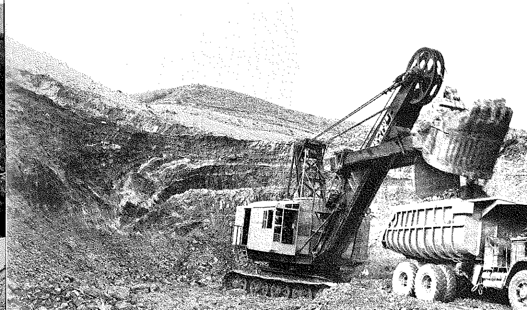
▼ Fig. 11. Excavating in elongated depression in top of porphyry sill, left abutment. Shows Morrison shale slumped into depression.
