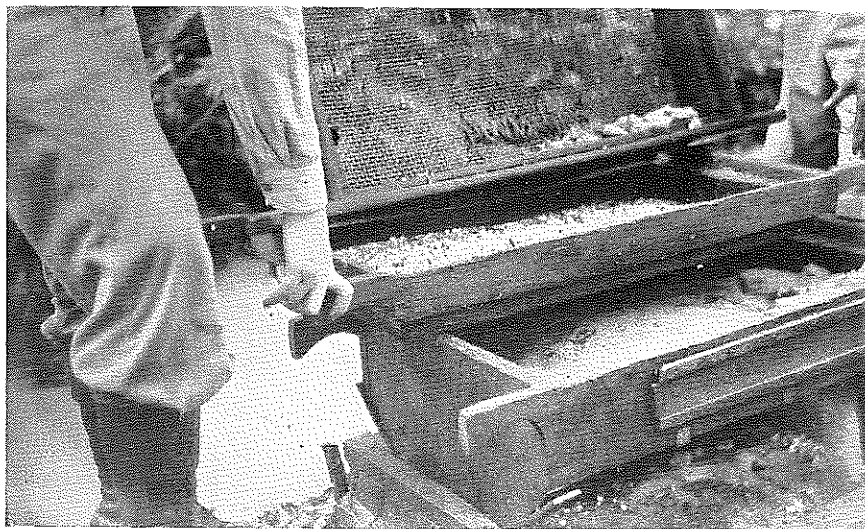
▼ Figure 2. Three Trays of a Diamond Shaker.
